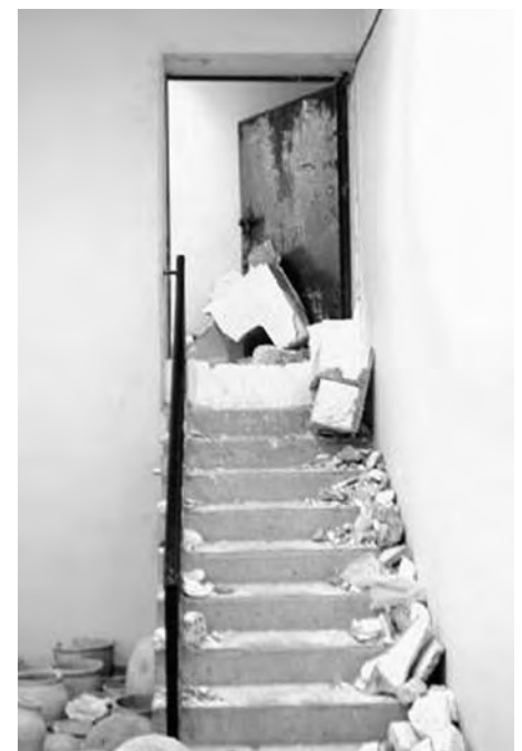
Figure 2. Museum officials attempted to secure the basement by blocking the doorway with a wall of cinder blocks. However, sometime between April 10 and 12, 2003, looters breached the doorway, allowing them access to areas in which some of the most precious artifacts were stored. Photo courtesy of McGuire Gibson
